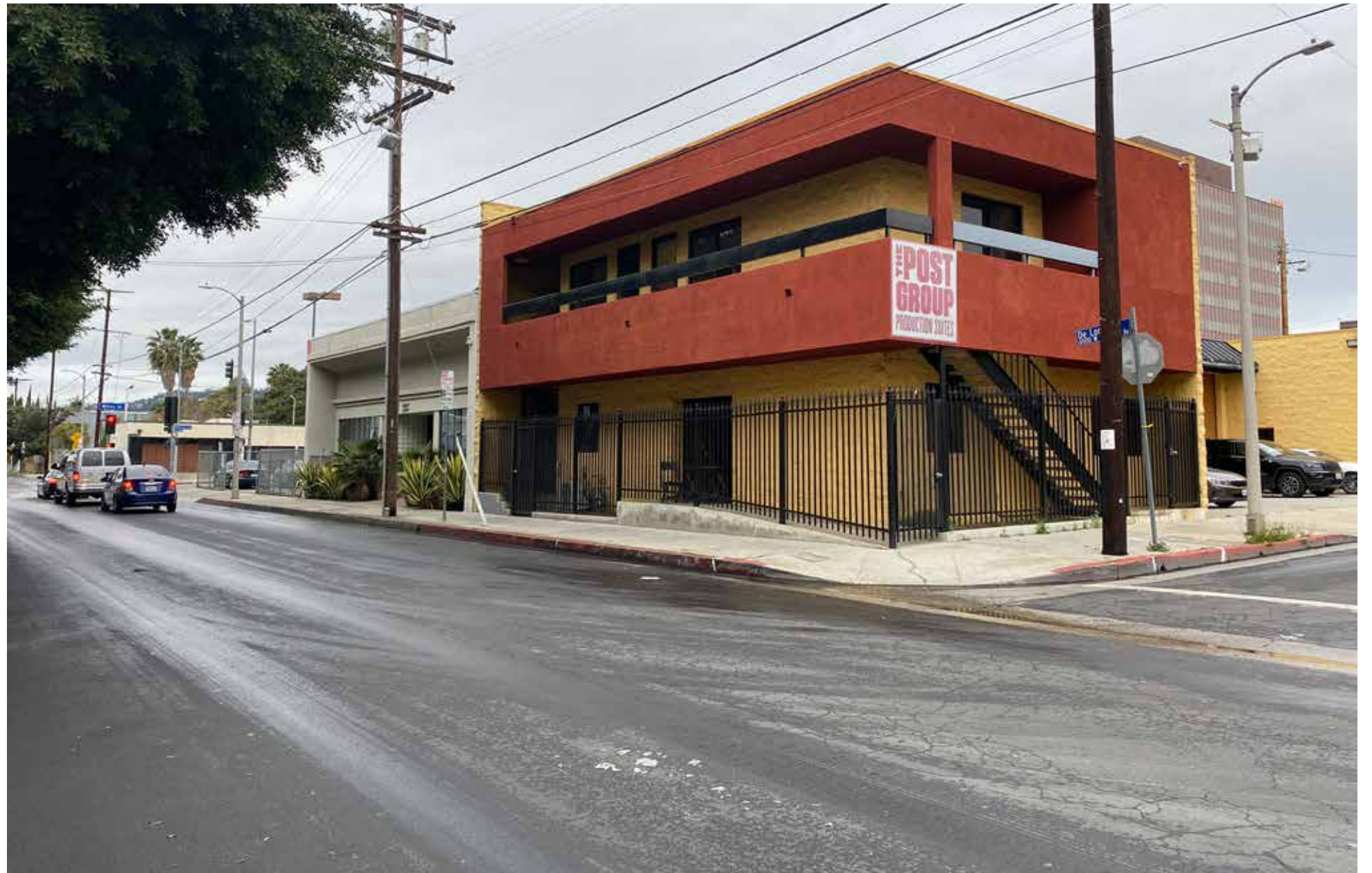
4 VIEW NORTH AND WEST FROM THE CORNER OF DE LONGPRE AND COLE
